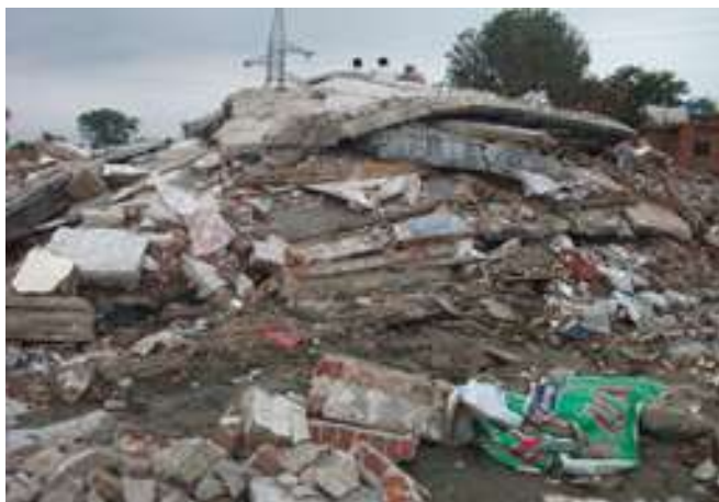
Rubble of a hotel in SWAT destroyed in Floods
