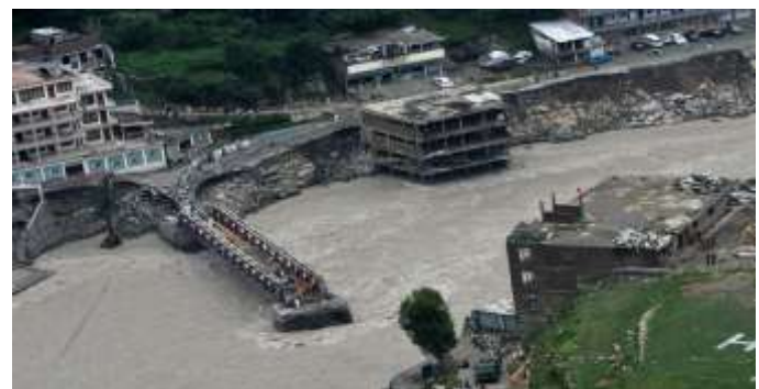
Damages in Khyber Pakhtunkhwa
